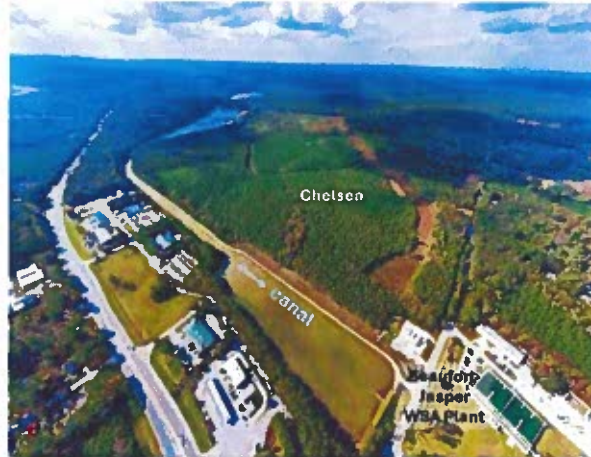
Chelsea's southern border buffers BJWSA's open-air drinking water canal. (Photo by Holstein Appraisals)
