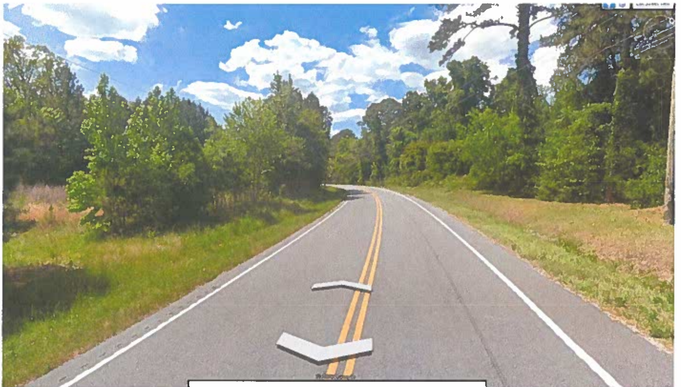
SC 462 – View Looking West from S-19 Intersection
